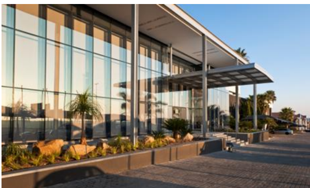
Completed solar installation at 130 Gazelle
