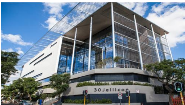
30 Jellicoe at 94% occupancy
