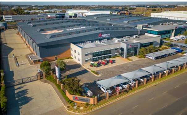
Completed solar installation at 16 Pamona
