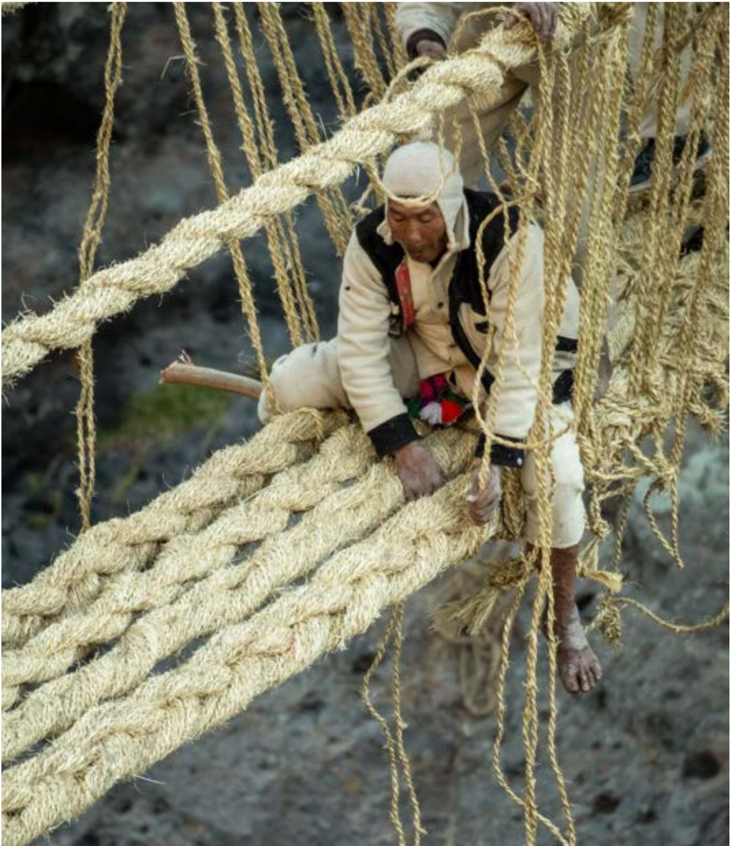
Bridge building at Q'eswachaca.
